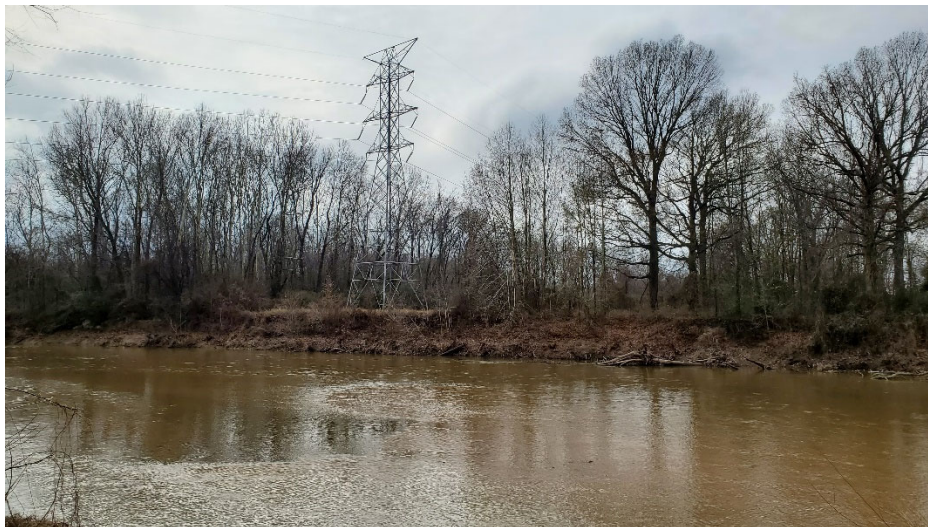
Figure 5. Streambank Erosion Adjacent to Tower #1613
