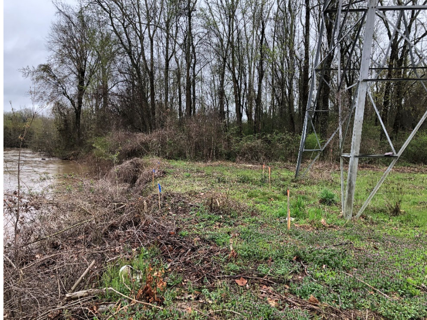
Figure 4. Streambank Erosion Adjacent to Tower #1613 Closeup
